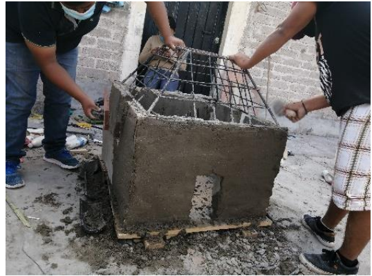
Fig. 6. In the figure you can see the disassembly of the sheer that was placed event to the concrete coating, to obtain a better aesthetics. Source: Photograph taken by the team.
