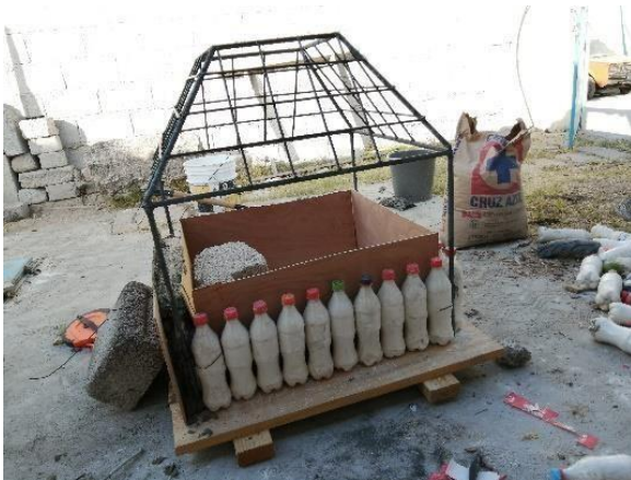
Fig. 4. The PET bottles are attached to the metaclie structure, placing a wooden mold to serve as a molding when pouring the concrete for its coating and better firmness. Source: Photograph taken by the team.
