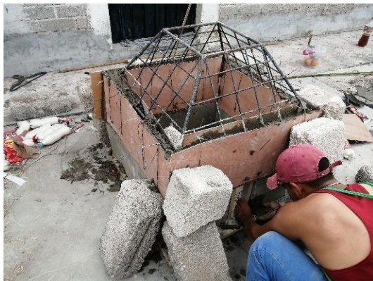
Fig. 5. Once all the PET bottles have been placed and once fastened, they are coated by means of concrete. Source: Photograph taken by the team.
